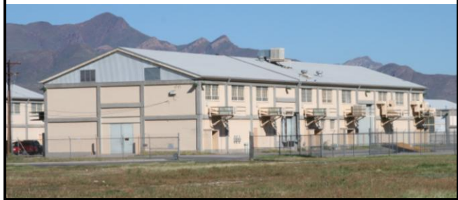
Figure 2-8: Building 1094. Eligible for inclusion in the National Register of Historic Places as the Universal Missile Training Building, SAFEGUARD Central Training Facility (1973-1975) along with the silos located adjacent, to the right.
